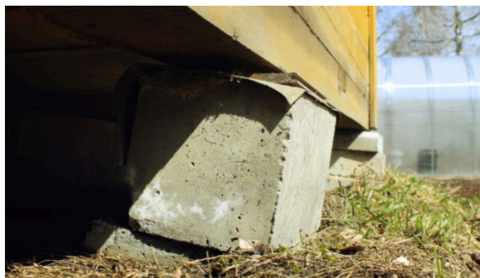
An inadequate base damages your shed.
