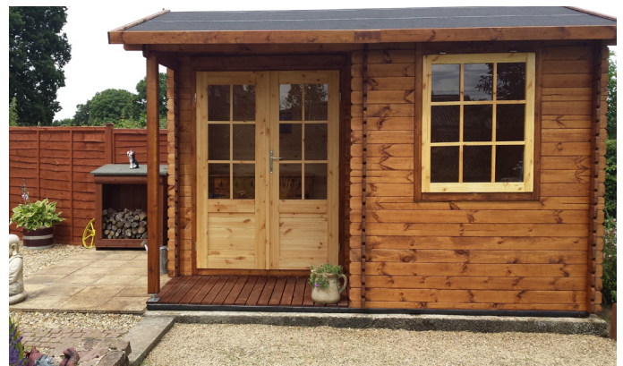
A solid concrete slab base is best for a heavier shed or log cabin.
