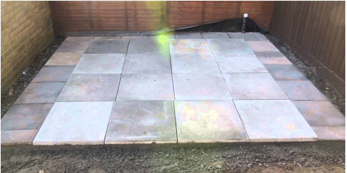
Paving slabs are a flexible option - either make just a shed base, or extend the area into a patio
