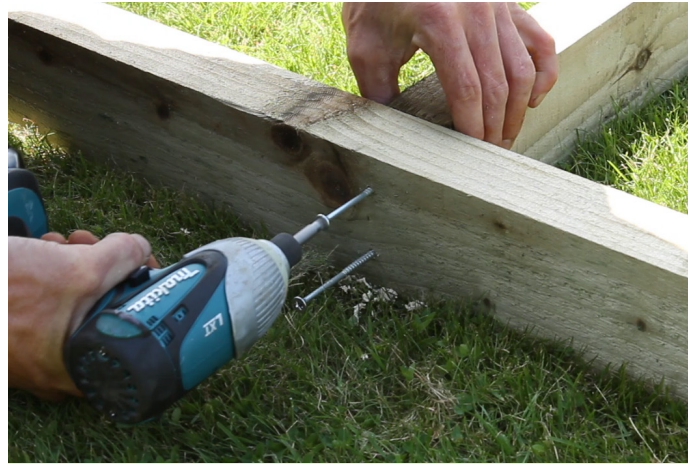
Screw the frame together.
