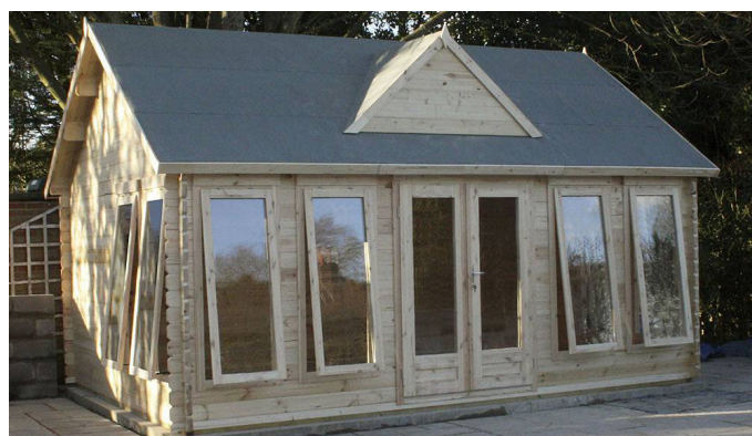
A larger building like this log cabin will require a sturdy, concrete base.
