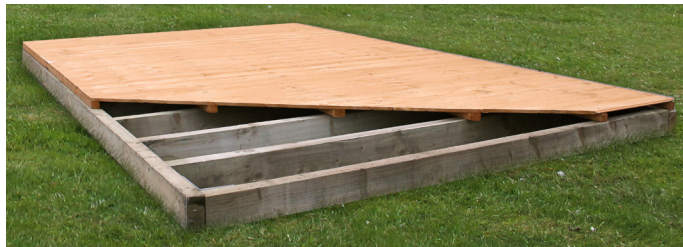
A fully assembled portabase with a shed floor installed.
