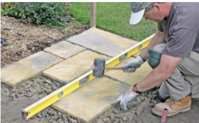
Use a rubber mallet to set each paving stone.
