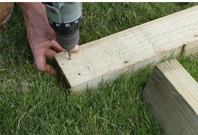
Pre-drill holes ready to screw the timbers together.
