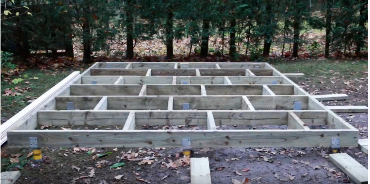
The StopDigging team install ground screws to support your shed base
