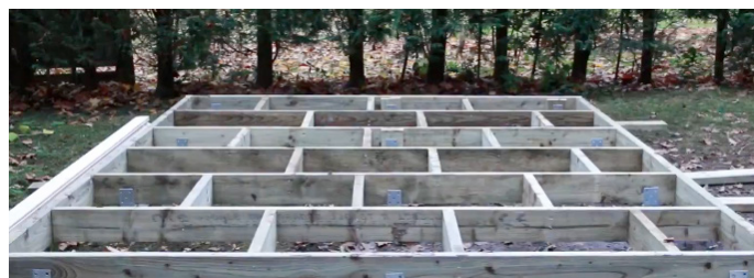
A StopDigging base is installed by dedicated professionals.
