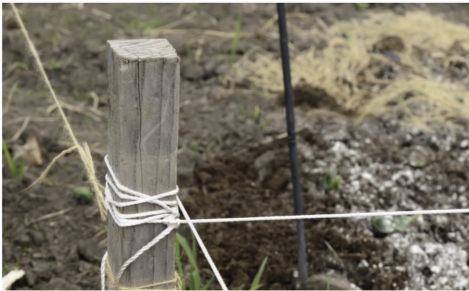
Keep measurements accurate and you'll have a better fitting shed base.
